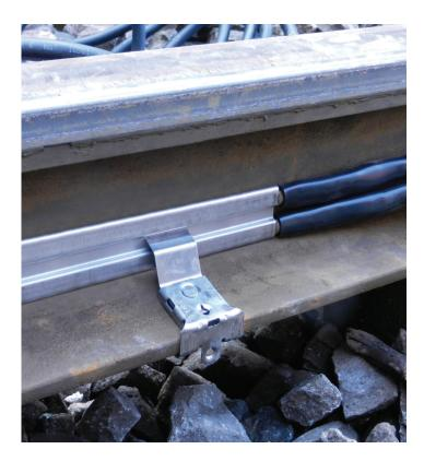
**BUS WIRES COLD AREA** SELF-REGULATING **HEATING CORE** JACKET
