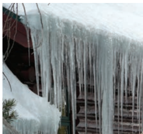
Unprotected roof and gutters
