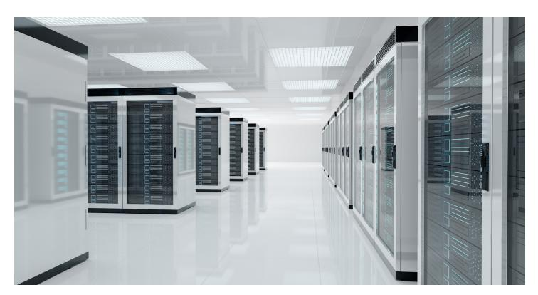
Perforated or mesh doors promote proper airflow to the equipment to prevent overheating and should be used to provide sufficient airflow, preventing overheating, and should be used on the front and rear of all server enclosures.
