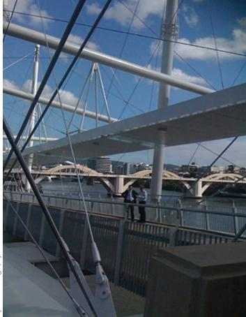
The Kurilpa Bridge is the world's first tensegrity pedestrian and cycle bridge.
